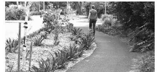
At-grade walking path behind green stormwater infrastructure without curb in the City of Shoreline.
