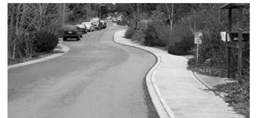
Traditional concrete sidewalk with curbs on one side of the street only, with rain gardens that could be implemented in coordination with Seattle Public Utilities. 2nd Avenue NE pictured above.
