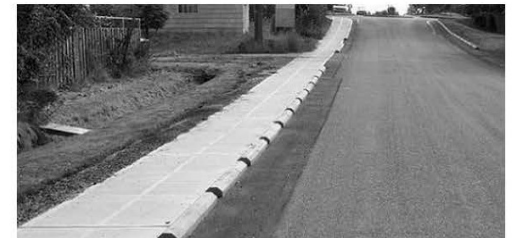
Curb-separated walking path at the same level as cars at N 97th Street and Fremont Avenue N.
